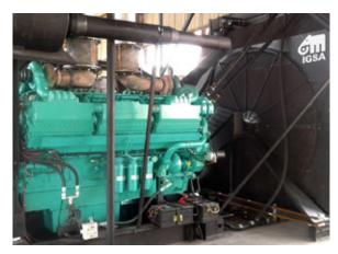
2 x 2.5MW generator sets help power the extraction site
