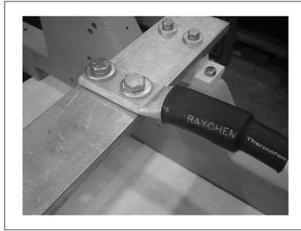
FIGURE 25. CORRECT CABLE CLAMPING
