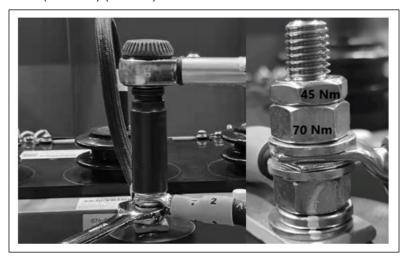
FIGURE 19. CORRECT CABLE CLAMPING (MULTIPLE CABLES)
