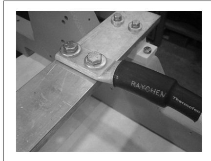
FIGURE 27. CORRECT CABLE CLAMPING
