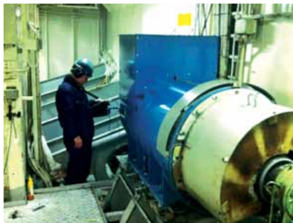
Inside the engine room with a new STAMFORD PM7
