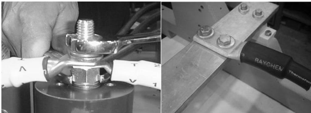
Figure 1: Showing the correct cable clamping methods.
