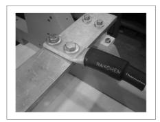
FIGURE 25. CORRECT CABLE CLAMPING
