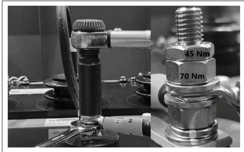
FIGURE 25. CORRECT CABLE CLAMPING (MULTIPLE CABLES)
