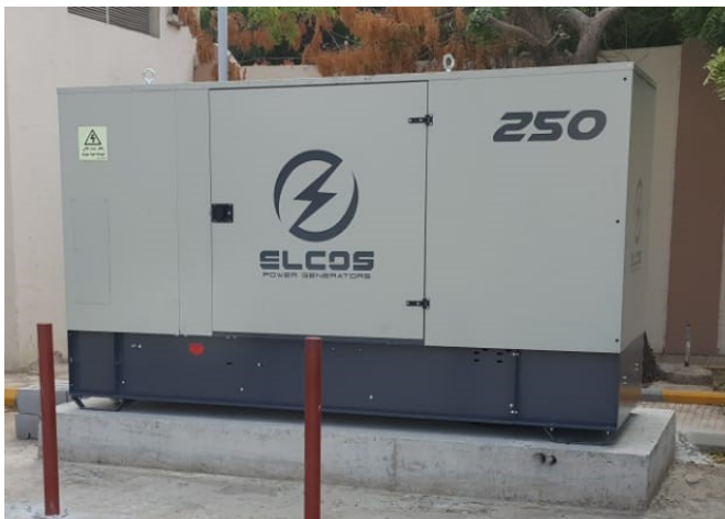
One of the four generator sets in situ at the hospital
