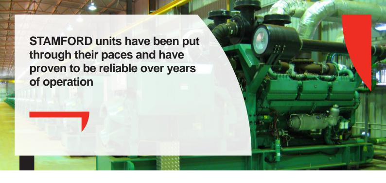
The latest of the three Western Australian mining projects is Christmas Creek, owned and operated by the Fortescue Metals Group. Situated in the state's Pilbara region, the iron ore mine has a 58MW prime power requirement, making it the largest of the three sites, and uses 28 high voltage STAMFORD P80 alternators. These alternators each have a 2,500kVA output and bar wound technology.
