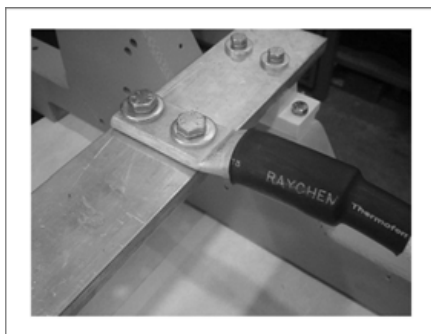
FIGURE 25. CORRECT CABLE CLAMPING
