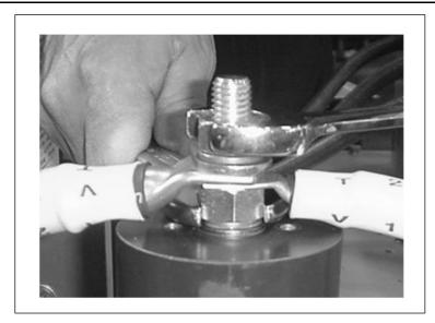
FIGURE 20. CORRECT CABLE CLAMPING (MULTIPLE CABLES)
