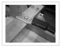
FIGURE 21. CORRECT CABLE CLAMPING (SINGLE LOAD CABLE)
